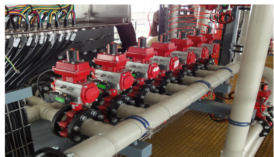
Fig. 3: Filtrate outlets including sight glass for each outlet. Outlets are grouped into headers with individual pneumatically actuated valves leading into the filtrate collector.
